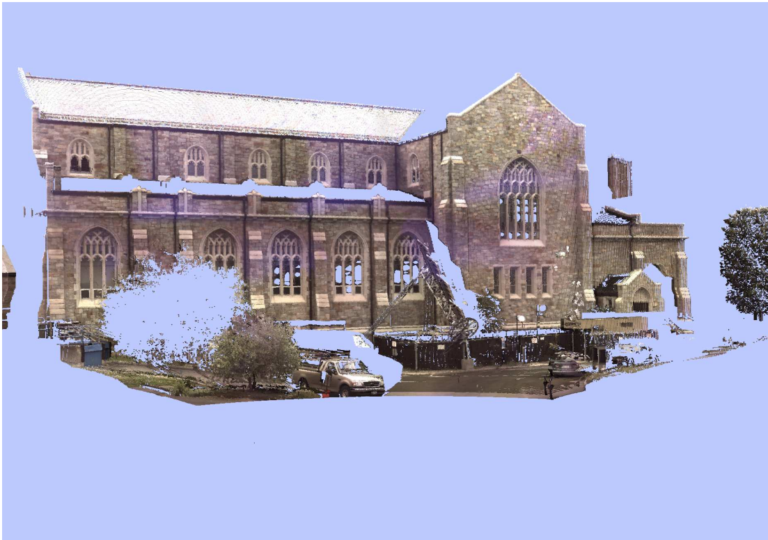
Figure 1.2: A LiDAR scan of a building. This scan contains 1.6 million colored points.
